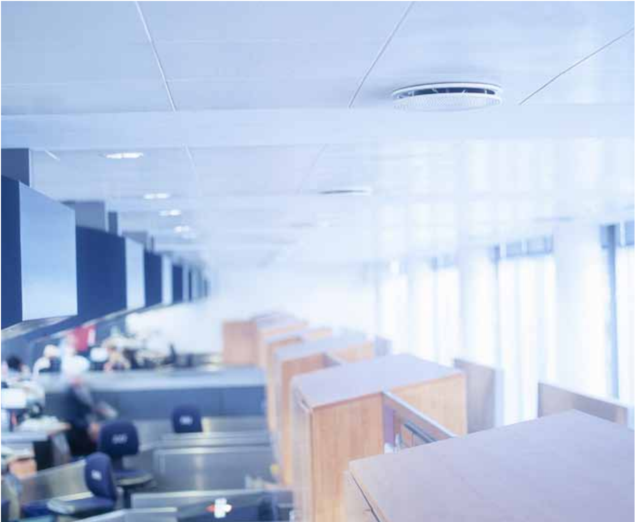
PCA, Terminal 3 - Copenhagen Airport
