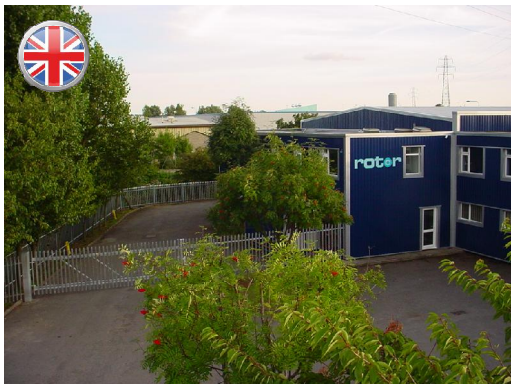
Regal UK 1,500m 2 facility is located in Wellingborough in Northamptonshire and distributes Marathon, Leeson and 'rotor' motors throughout the United Kingdom and Republic of Ireland.
