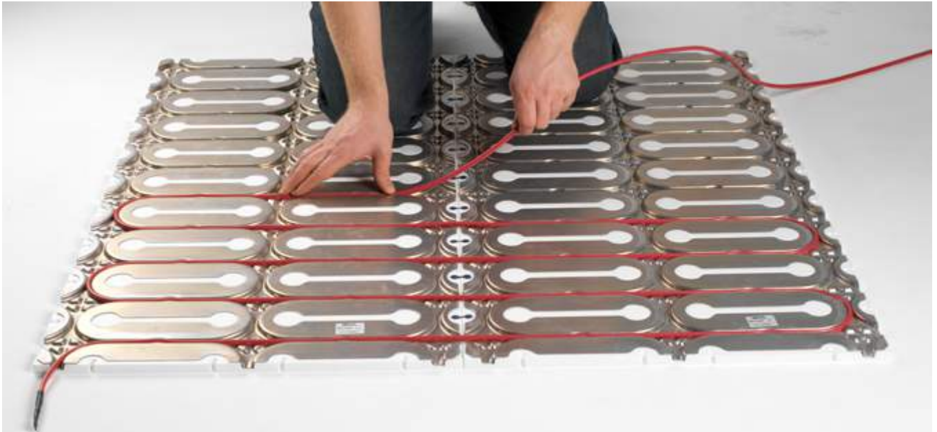
Fig. 20. Mounting method for heating cable into Reflect insulated plates (EFCI Dry)
