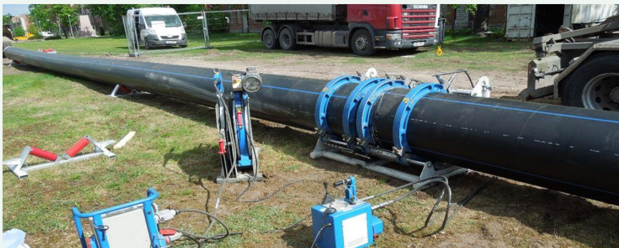
Figure 1. HDPE pressure pipes installation process stage
