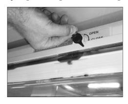
Remove the rubber protection on the central lock switch. Turn the central axis 180° to the left (marking - OPEN) with a socket wrench. Sliders release transparent cover and the lamp opens. When closing follow the orders of operations in reverse.
