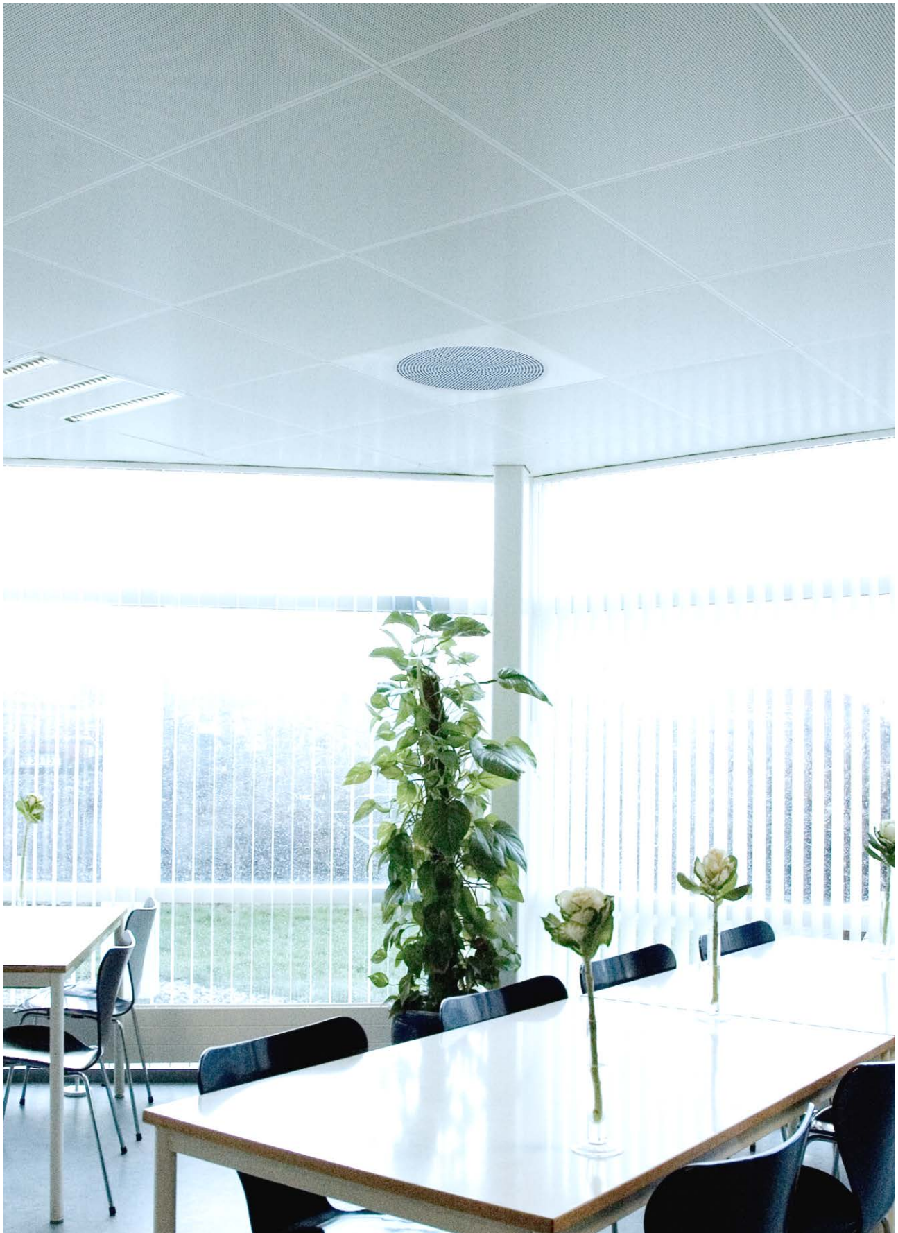
PC7, Integrated in Luxalon Clip-In ceiling with adapted module plate type LM.
