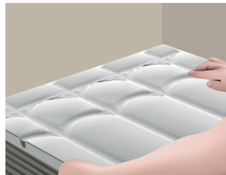
Adhering EPS board to the concrete substrate
