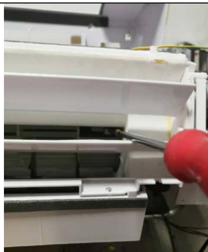
12. Loosen the screw at the motor shaft to take out the fan motor, then remove the motor to replace it.
