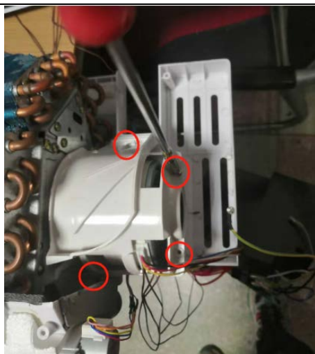
11. Loosen the screws at the motor cover
