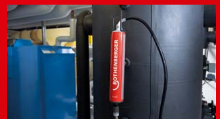
Set in size S with wall bracket and filling hose for the right station for demineralized water
