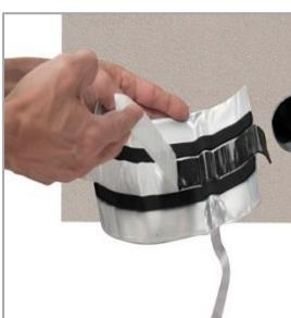
4. Apply lubricant on both OKT bag sides and on cable sheath
