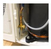
An additional Schraeder connection is fitted on the liquid line below the filter drier in the compressor chamber. It is also possible to use this connection for charging or servicing.
