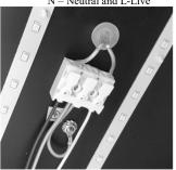
4. through small holes in the fixture, thread the wires
